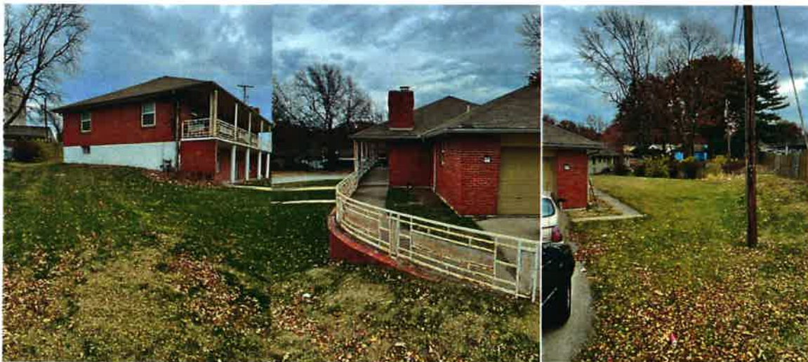
Figure 1 – Site Photos. East side. West Side with Ramp to second floor. Back Yard.
